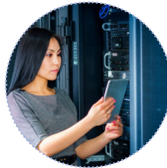
Training for Implementation and Support Engineers
